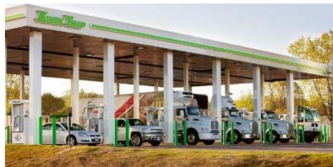
Public fast-fill CNG station. ANGI
