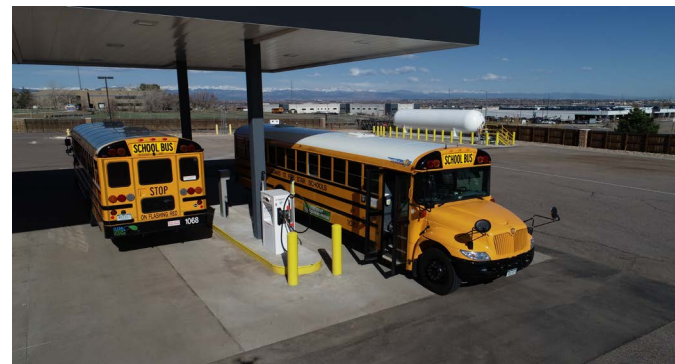
18,000 Fuel tank with dual two hose dispensers. Adams 12 School district
