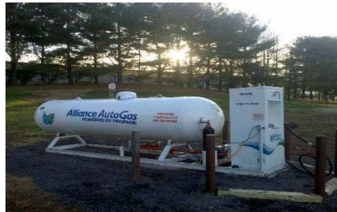
Skid-mounted 1,000-gallon storage tank and dispenser. Blossman Gas, Inc.
